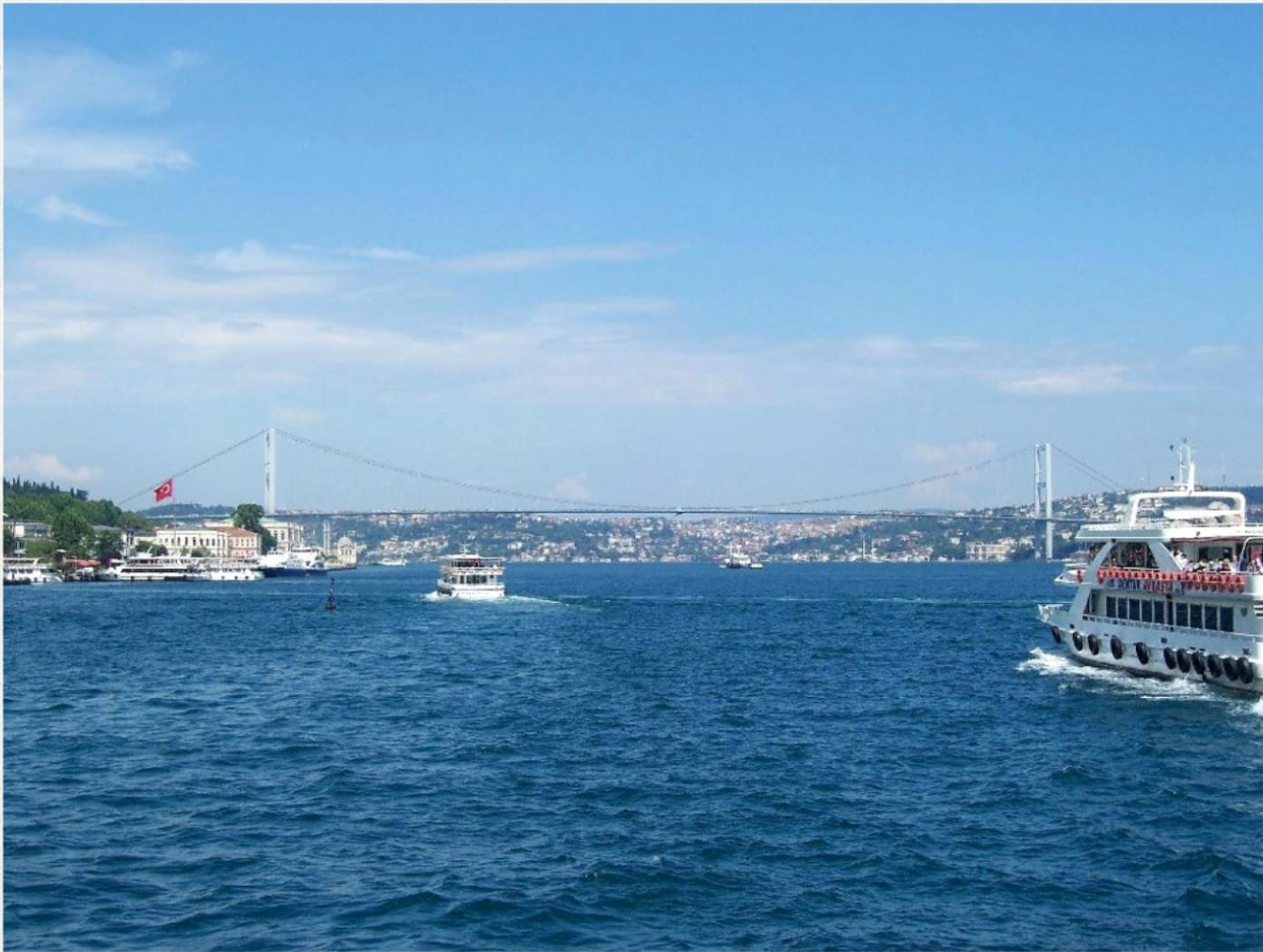
The bridge in the distance connects Europe (left) and Asia (right).
