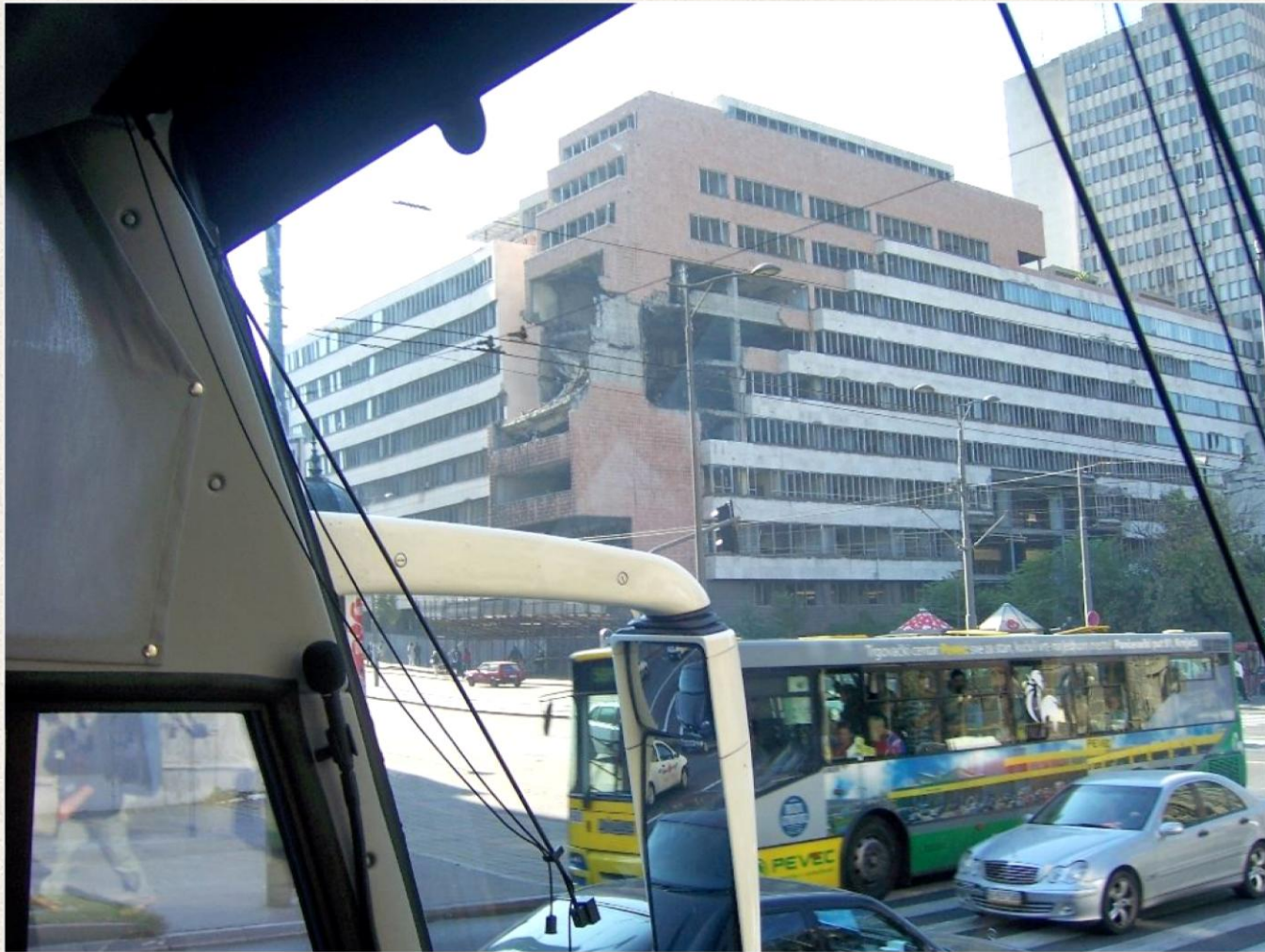
In Belgrade, Serbia, this is one of the buildings damaged during Bill Clinton's 78 days of continuous cruise missile attacks.
